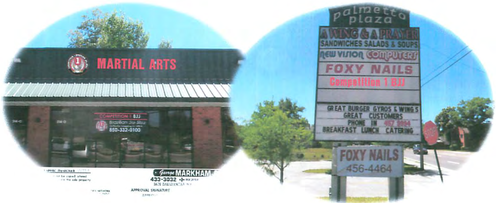
Installation of new signs 314 South Navy Boulevard
